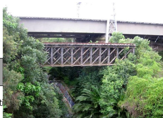
The original Whipple Bridge constructed in 1886 at Lewisham
